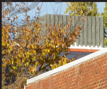
Example of appropriate roof-mounted HVAC screening.
